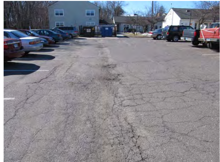
Asphalt-paving exhibits significant wear and deterioration
