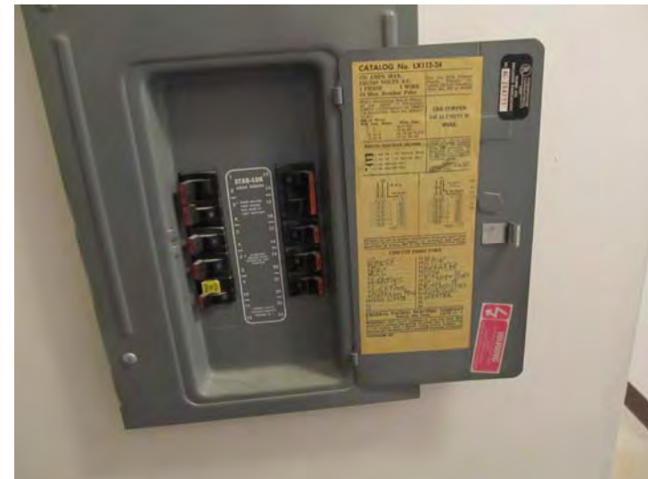
Typical Stab-Lok by FPE circuit breaker panel found at each unit
