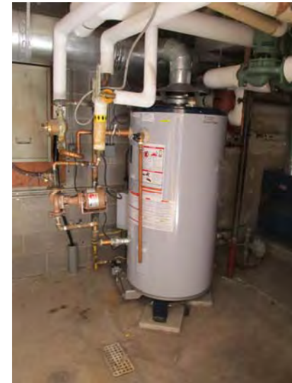
Typical, freestanding, natural gas-fired domestic hot water tank found at each residential building
