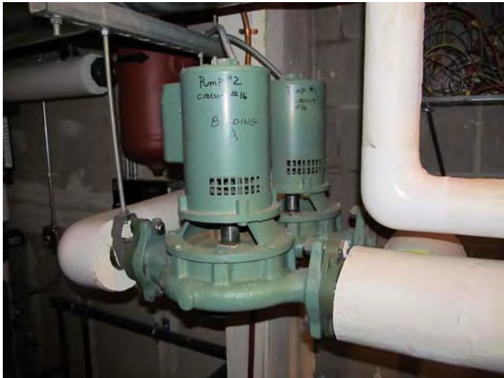
New pumps for circulation of hydronic heat installed concurrent with new boilers
