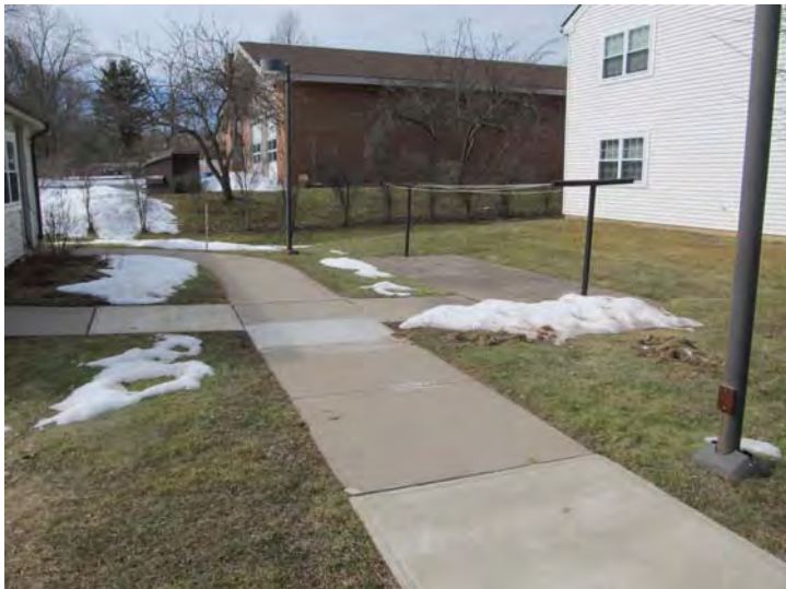
Typical concrete sidewalk with areas of past sectional repair evident
