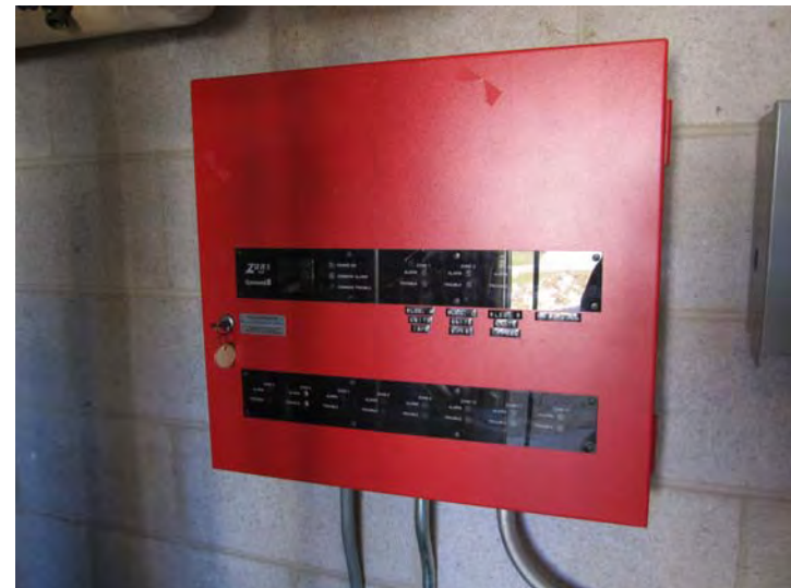
Central, zone-type, fire alarm control panel – Serviceable but at end of expected useful service life
