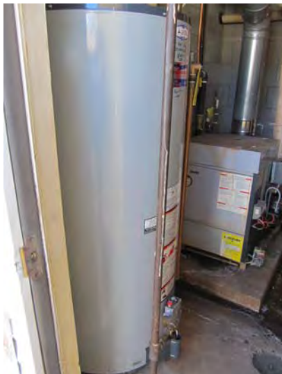
Boiler for hydronic heat production and freestanding domestic hot water tank that serve community building
