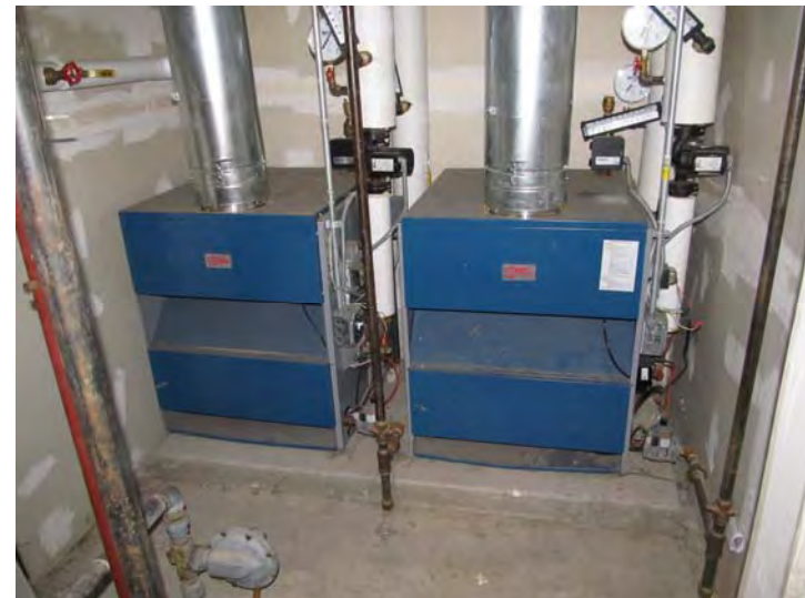
Typical, recently installed, natural gas-fired boilers found at each residential building
